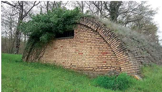
Figure 2. Old aqueduct at Tre Croci, Vetralla (VT), Italy
