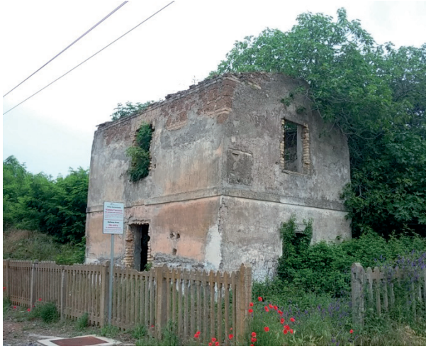
Figure 3. Railway cabin on the Rome-Viterbo railway line
