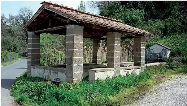
Figure 18. Public washhouse, Tobia (VT), Italy
