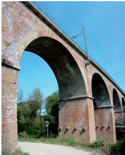
Figure 13. Railway bridge along the Rome-Viterbo line.
