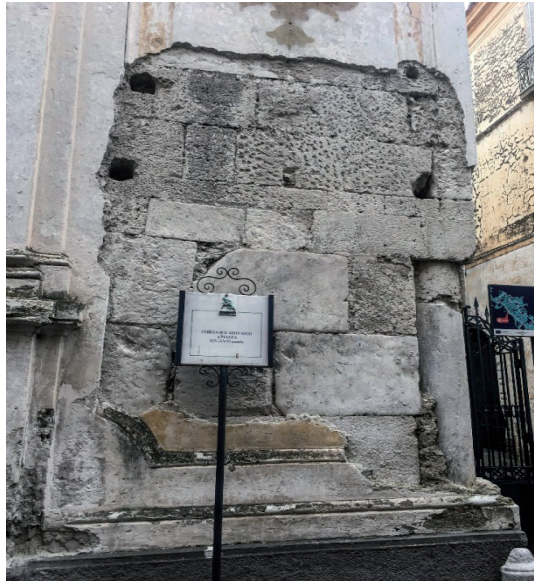
Figure 4. Sessa Aurunca (Caserta), Church of San Giovanni in Piazza. The portion of façade (right side) is useful for understanding the revealed masonry composed of blocks of reused limestone with a corner column and superimposed rows of ashlars making use of grey Campanian tuff (photo: Cesare Crova).
