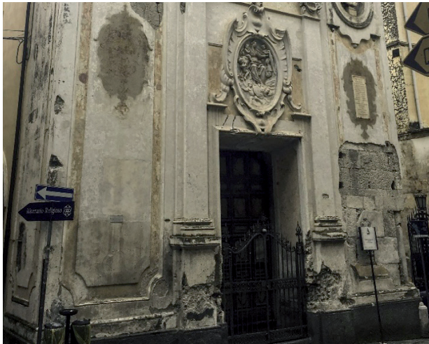
Figure 3. Sessa Aurunca (Caserta), Church of San Giovanni in Piazza. The base object of the thermographic investigation. The portion on the left is substantially intact, although marked by evident decay of the material; the portion on the right highlights a large gap in the plaster (photo: Francesco Miraglia).
