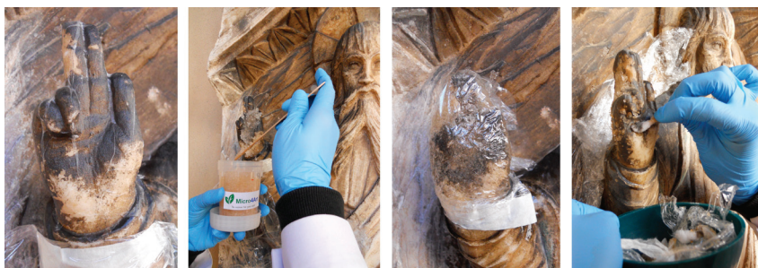
Figure 3. Bioremoval: (from left) before processing; Japanese paper and gelled solution application; covering by transparent polyethylene sheet; black crust removal.
