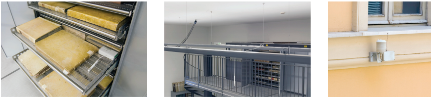
Figure 3. Position of sensors a) inside cabinet b) inside repository c) outdoors
