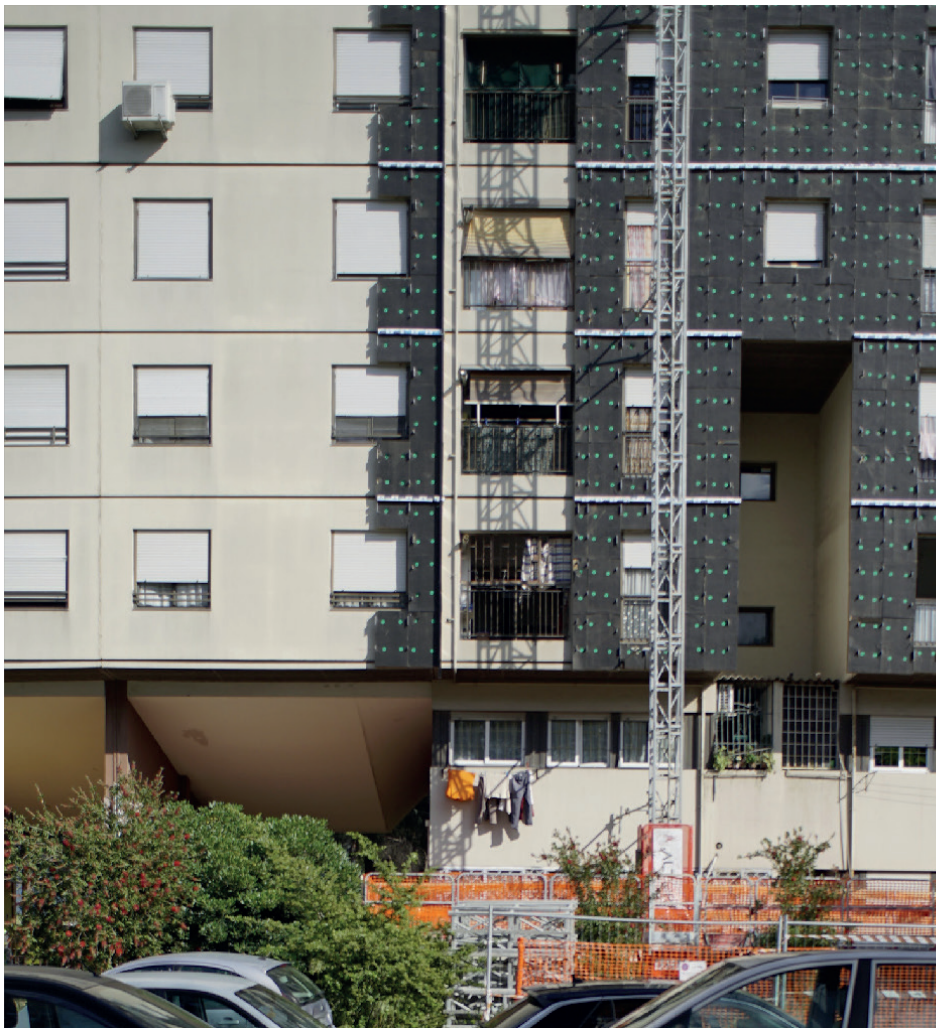
Figure 4. On-site view of envelope renovation: performance upgrade through a controlled rewriting of the original modular scan. Credits: Vannini, C. 2025.
