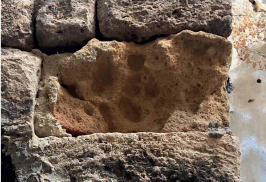
Figure 10. Deterioration and exfoliated sandstone, melted and deteriorated under the effects of acid rain (Source: Authors, 2023).
