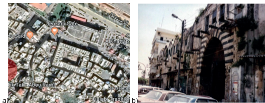
Figure 5. The old Mameluke commercial building. a) Location; b) façade.
