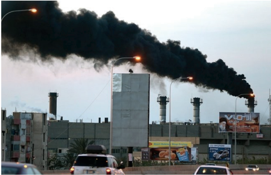
Figure 2. Jiyeh power plant (Source: AZAKIR, 2013)
