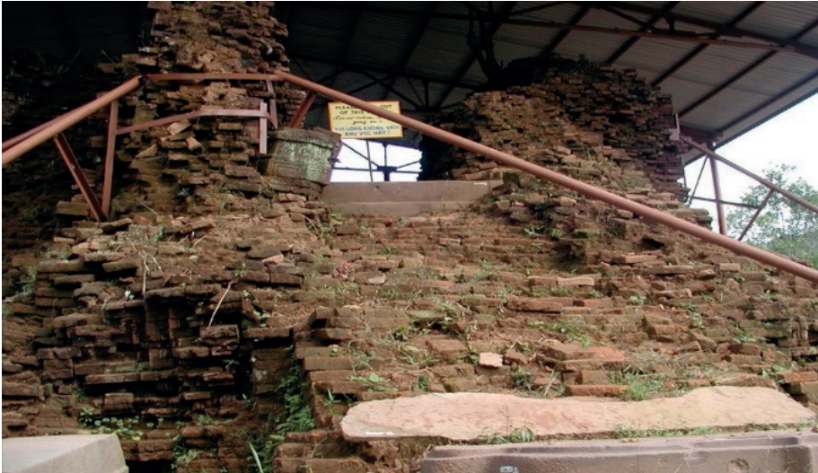
Figure 3. The F1 tower at My Son in Vietnam is at risk of collapse. Photo by Nguyen Quang Hieu.
