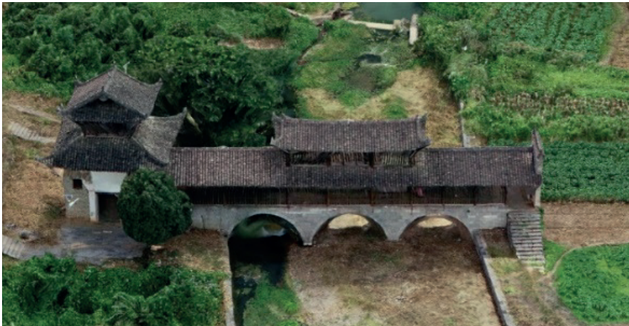
Figure 2. Aerial view of the Huilan wind-rain bridge
