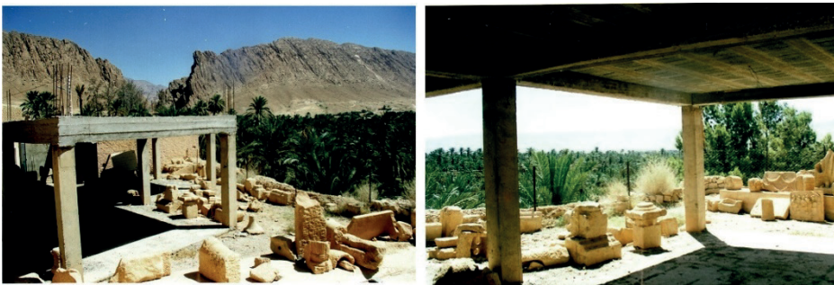
Figure 15. Reinforced concrete structural system of the Lapidaire Museum before its demolition/reconstruction.
