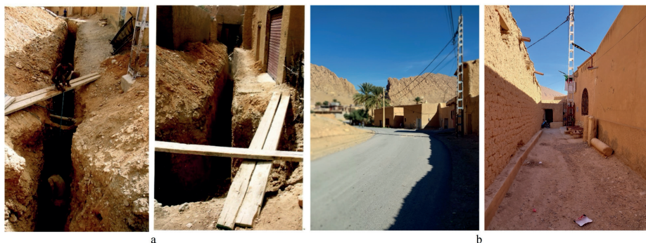
Figure 14. Infrastructure renovation: a) Before renovation; b) after renovation.
