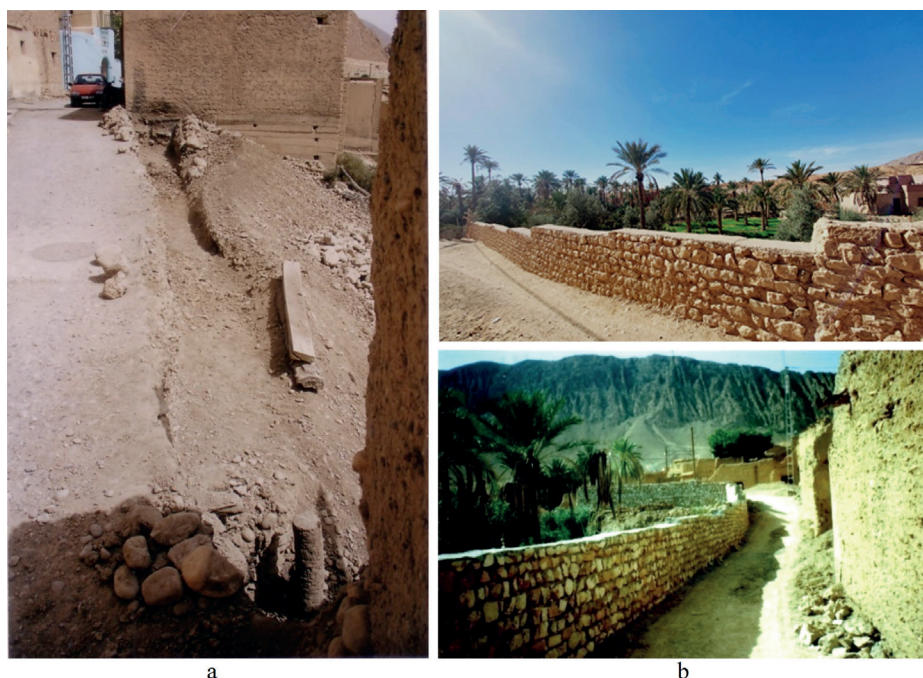
Figure 13. Views of the boundary walls: a) before renovation; b) after renovation.
