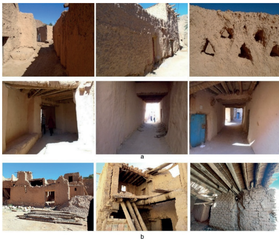
Figure 6. Current views of Dachra El-Hamra, El-Kantara: a) Façades and passageways; b) traditional building materials.
