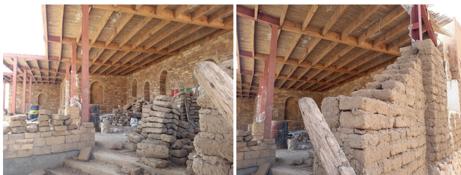
Figure 16. Lapidaire Museum during its reconstruction using compatible materials.
