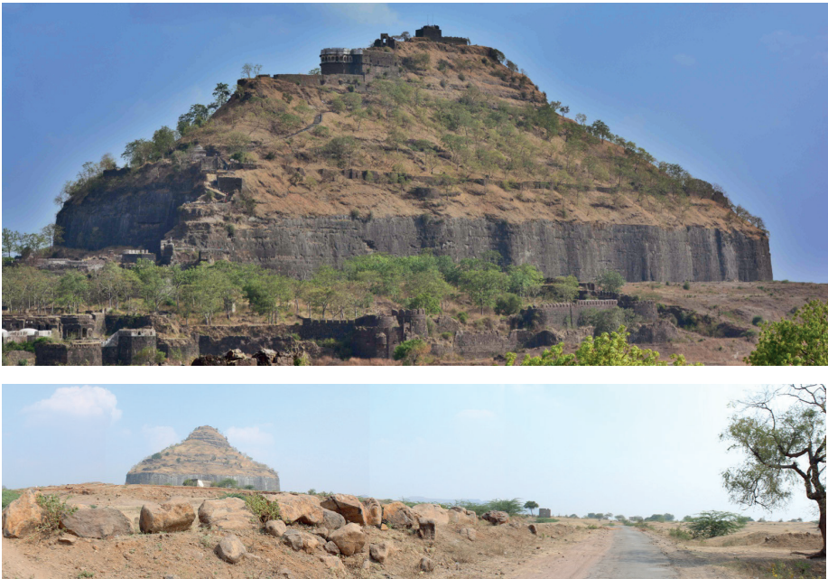
Figure 5. Rear view: core hillock of Daulatabad fort.
