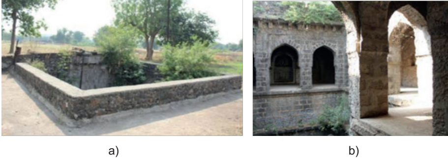
Figure 12. a) The well in the farmland setting; b) the space inside with structures around the water.
