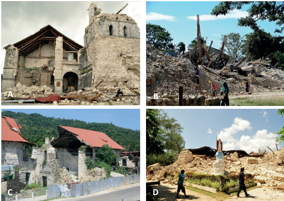
Figure 10. Damaged coral stone structures of Bohol. (A) Baclayon Church; (B) Loon Church; (C) Loboc Church; (D) Maribojoc Church (Source: Wikipedia).
