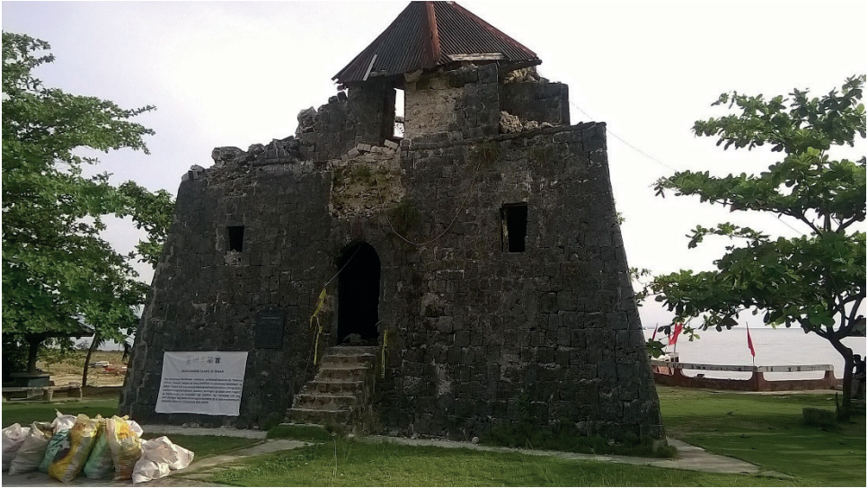
Figure 11. Damaged Punta Cruz Maribojoc watchtower (Source: Wikipedia).
