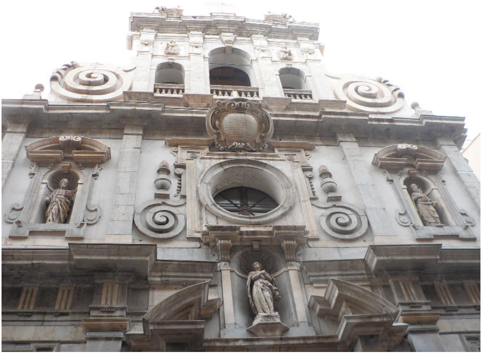
Figure 2. Outside view of the Church of Saint Matthew (Pa).
