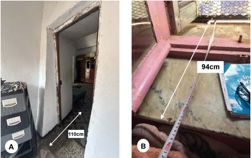
Figure 6. Metric measurements revealing the thickness of the wall. A) The base of the doorway; B) window width (source: Author, 2024).
