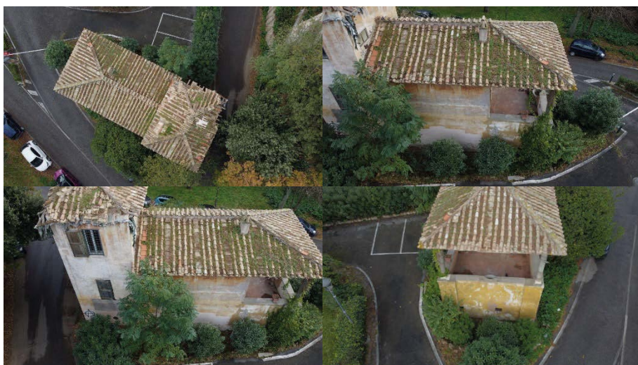
Figure 10. Aerial photos of the structure; damage to the roofs is clearly visible.
