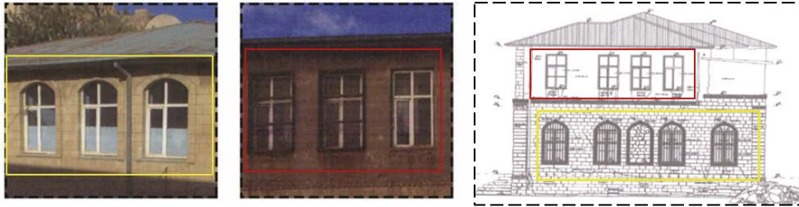
Figure 15b. The window types on the west facade were added to the ground floor in 1964 (highlighted in yellow), and the window types added to the first floor on the east facade in the 1990s (highlighted in red) [4].
