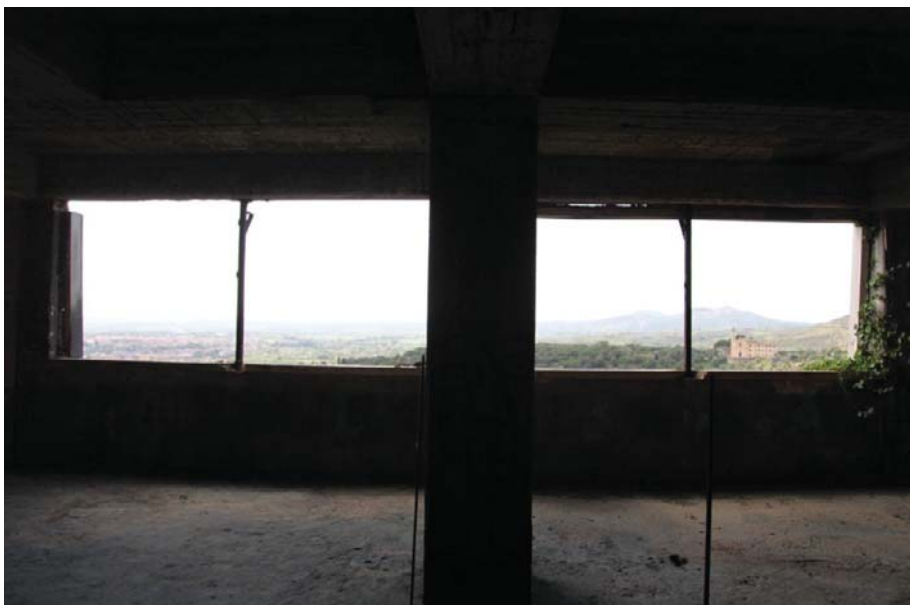
Figure 8. Image taken on the floor at 199 meters asl: that is the view from the facade facing the Aniene valley, towards the complex of the Sanctuary of Maria SS. Del Quintiliolo, on the right (Source: Carlo Vannini).
