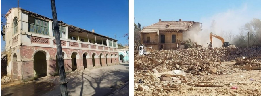
Figure 4. Demolition of the Sahara Hotel in 2023 [16].
