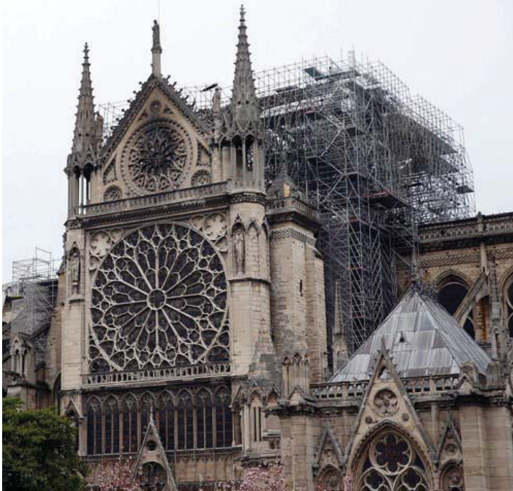
Figure 2. Cathedral restoration process after the fire in 2019.
