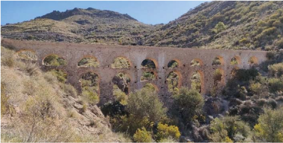
Figure 3. Current conservation state of the aqueduct.
