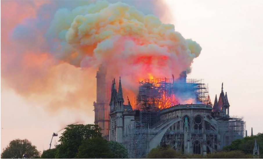
Figure 6. The collapse of the spire of Notre Dame Cathedral during the fire that broke out in 2019, occurred during an extensive restoration programmed for the church [36].
