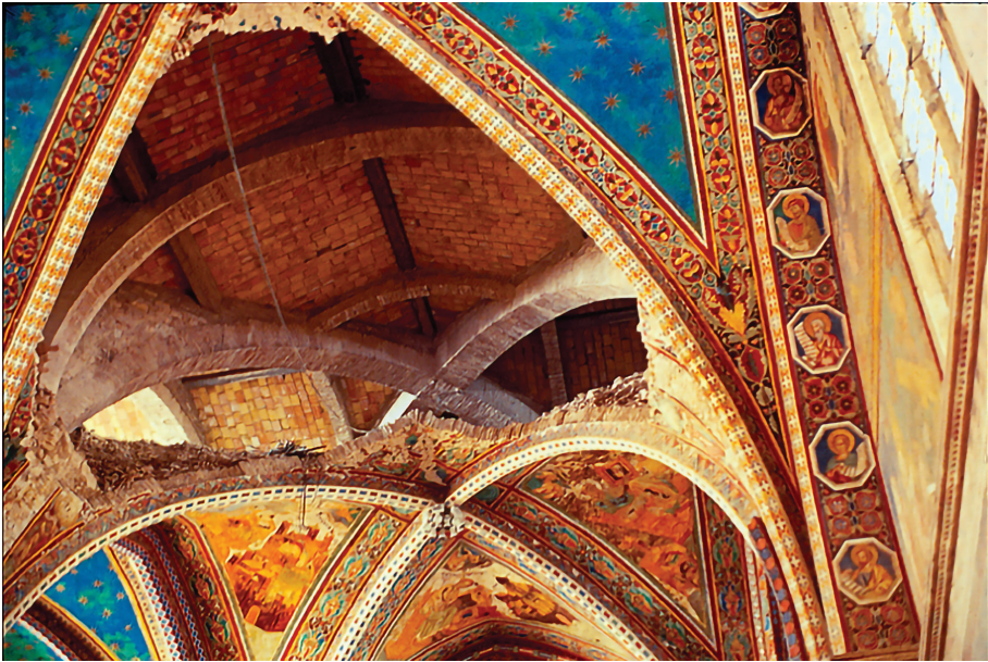
Figure 4. The collapse of the fresco ceiling in the Basilica of Saint Francis in Assisi following the 1997 earthquake [29].
