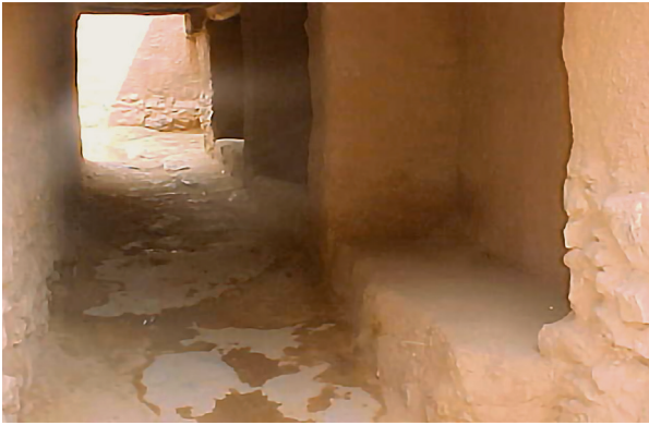
Figure 8B. Photo of the djemaa of the Taghit ksar [16].
