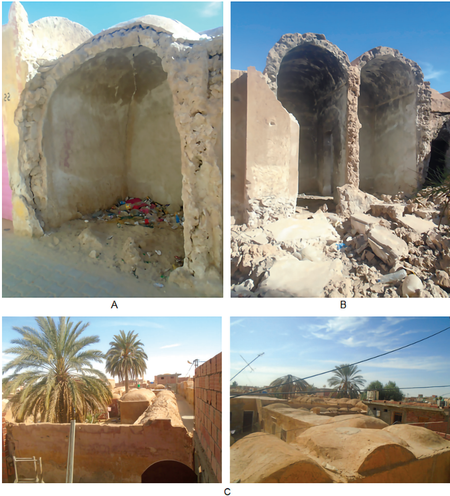
Figure 5. Current view showing the construction system in the Souf: A) and B) cross-section views of a dome and two adjoining barrel vaults supported on load-bearing walls; C) current views of houses in Gemar (Source: authors, 2022).
