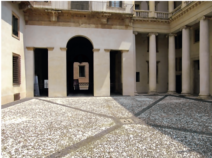
Figure 4. Courtyard of the Palazzo Barbaran da Porto (Vicenza, Italy). Source: Javier Pérez Gil.
