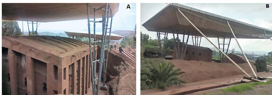
Figure 1. A) A canopy installed at the church of Bete-Medhane-Alem; B) the Bete-Mariyam Church with canopy.
