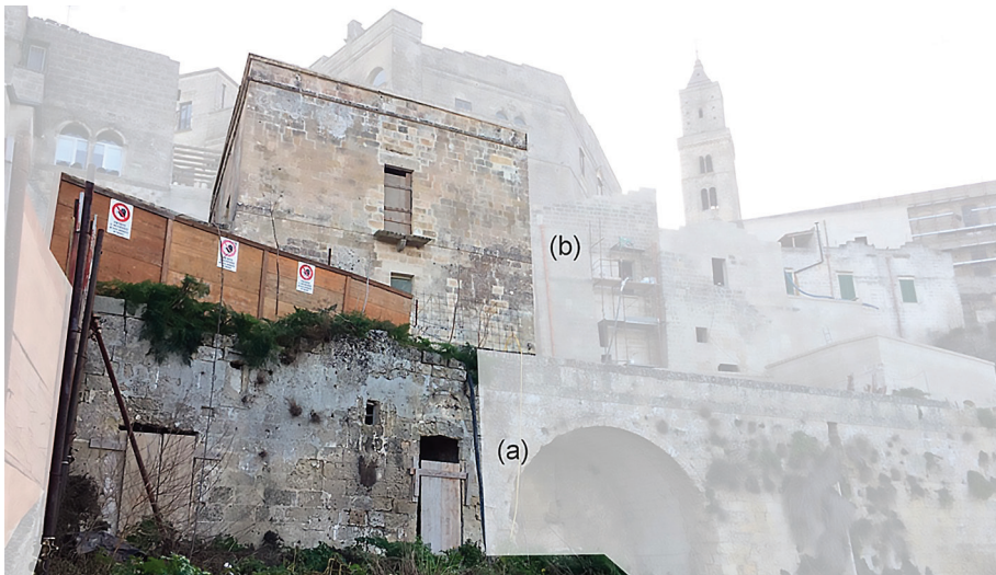
Figure 5. Image of the façade of the church (a) and its surrounding context, including Palazzo de Vitis (b).
