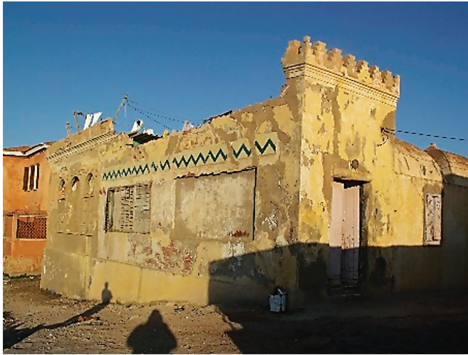
Figure 11. Villa A. Pommert, built in 1924 in Mostaganem; (source: Author, 2015).
