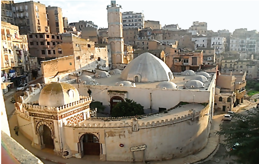
Figure 5. Pasha Mosque (source: Author, 2016).
