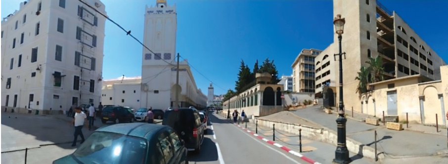
Figure 6. To the right stands a gigantic multi-storey car park in place of a square which gave an opening onto the Mosque.
