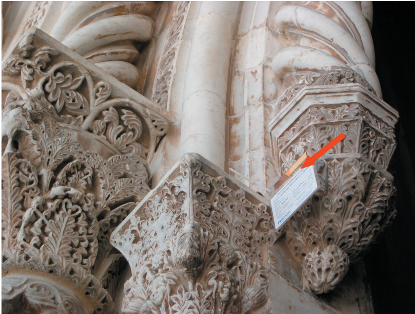
Figure 21. Positioning on the entrance gate of the cathedral.
