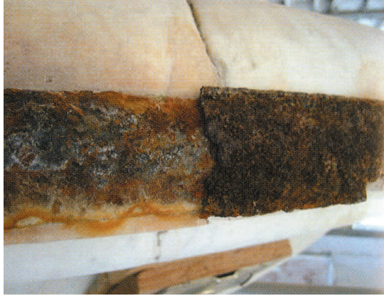
Figure 3. Chromatic alteration of the stem basin caused by the old metallic reinforcement rings [9].
